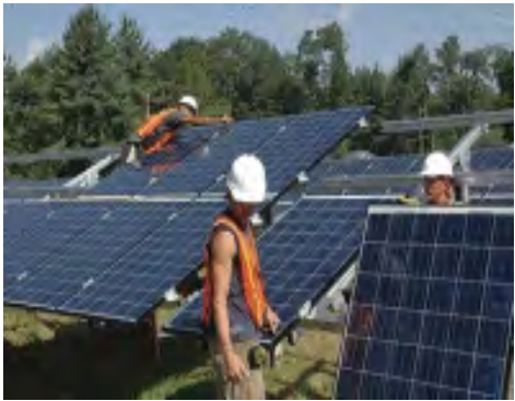
Specially trained workers install state-of-the-art solar panels.
